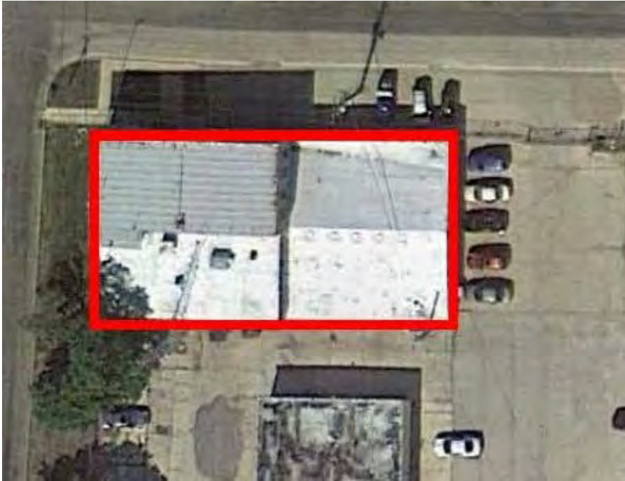
Old Sheriff's Building Pave lot after building demolition
